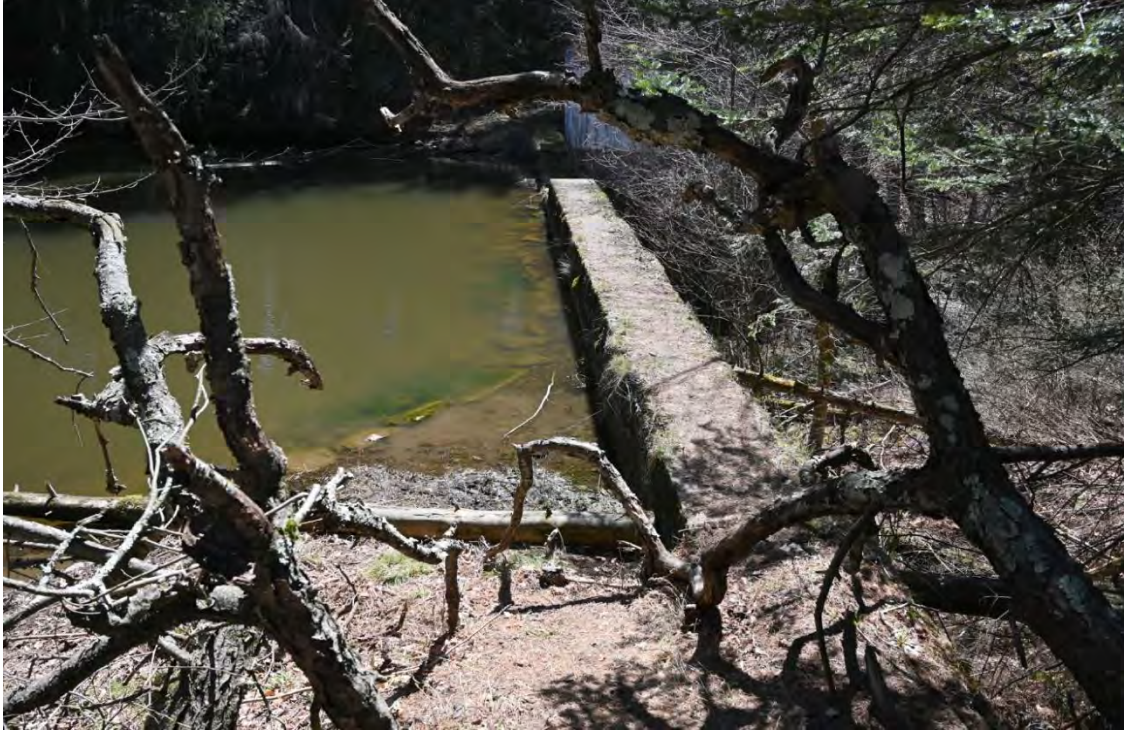
Figure 56. View of the upstream stone pavement feature, looking eastwards.
