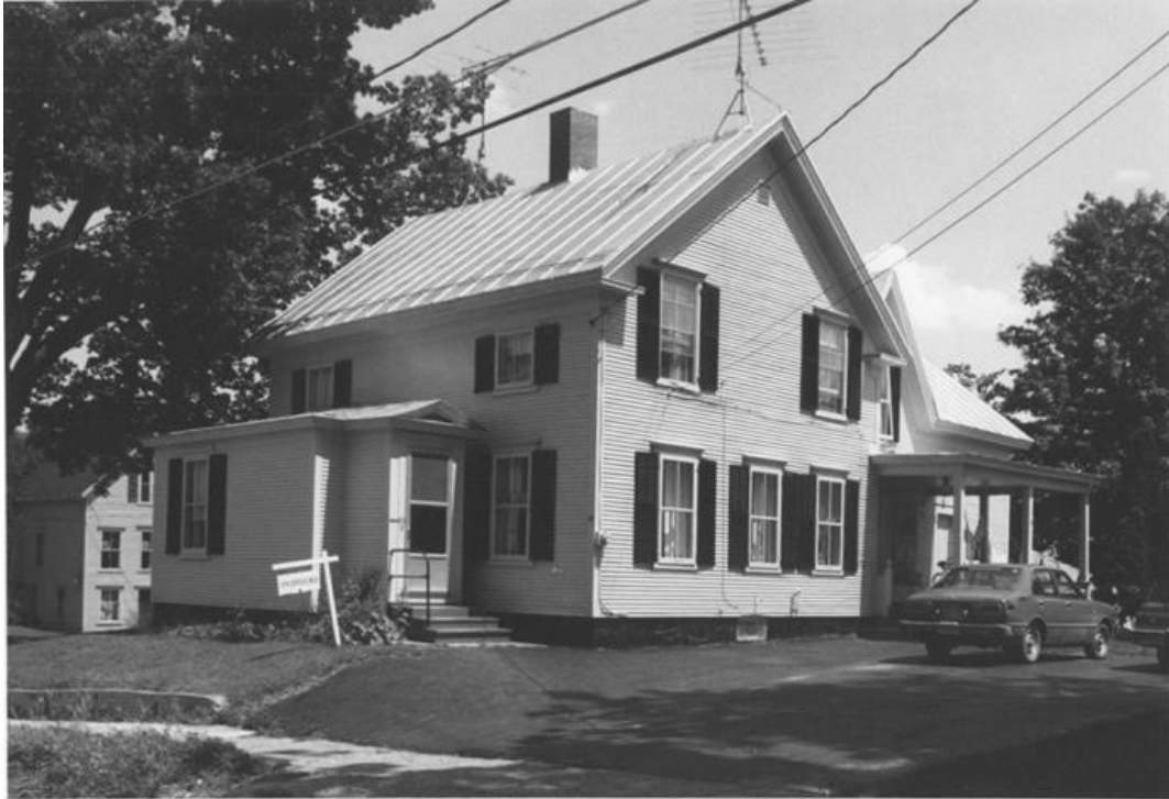
Figure 91. View northeast of the house at the corner of Bismark and Church streets (1984).
