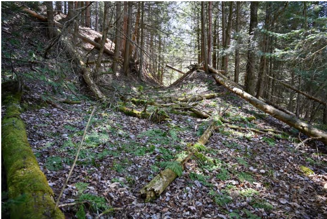
Figure 11. View of a former access road cut into the hillside at the left end of the dam, looking south.
