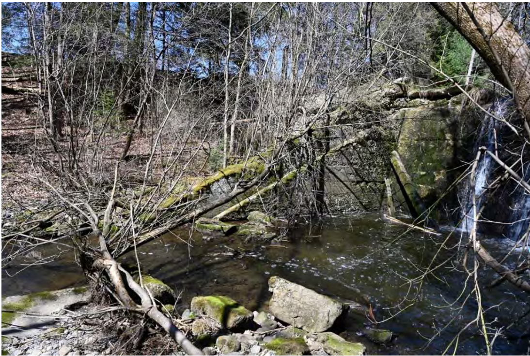
Figure 44. View of the spillway and apron area, looking west.
