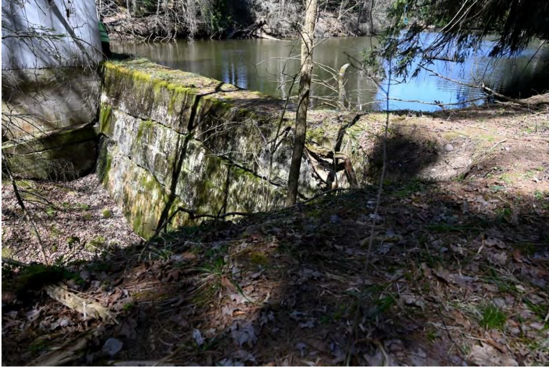
Figure 40. View of the right side of the main dam, looking west.
