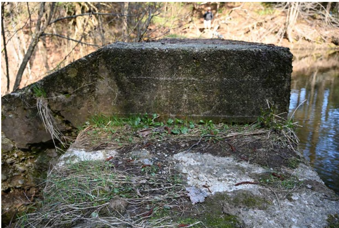
Figure 42. View of the right side of the spillway crest, looking west.
