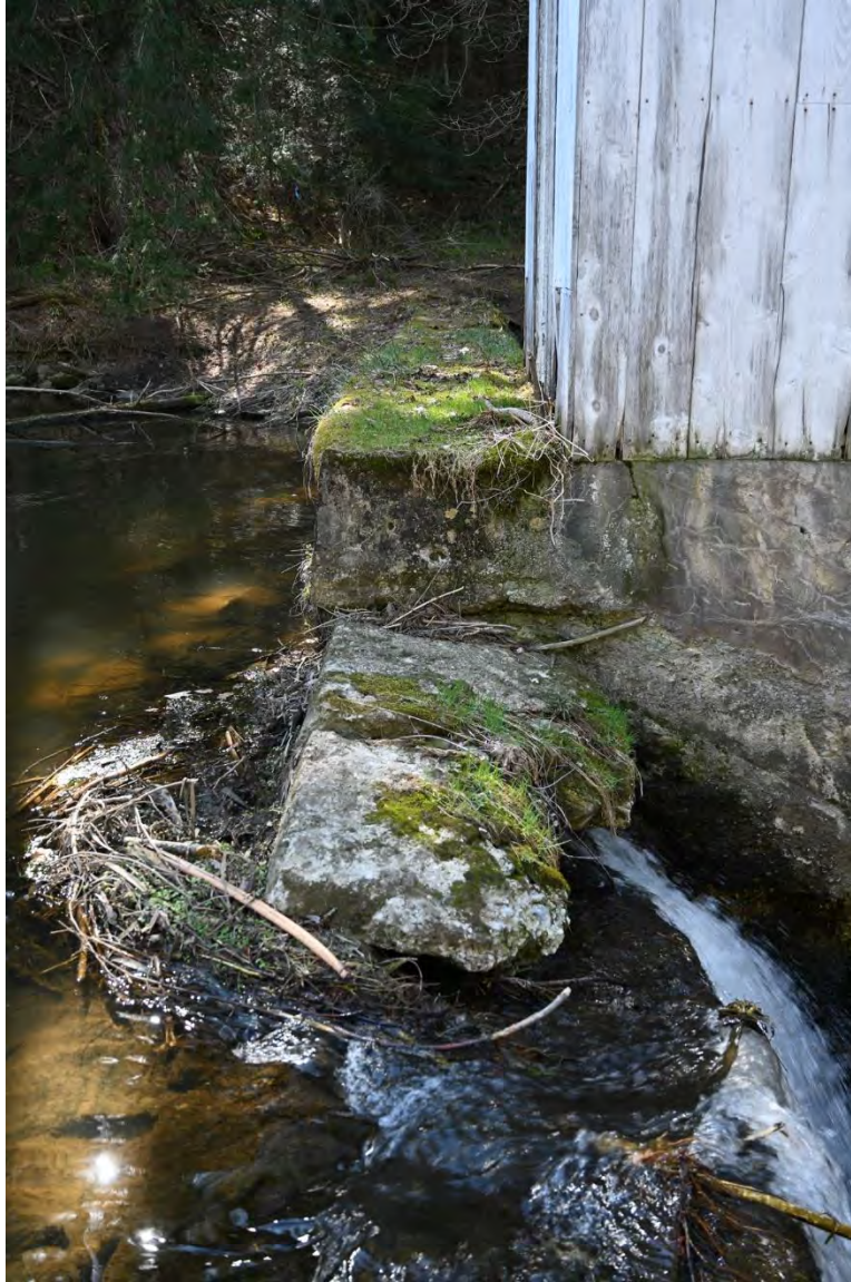
Figure 41. View of the right side of the spillway crest, looking east.
