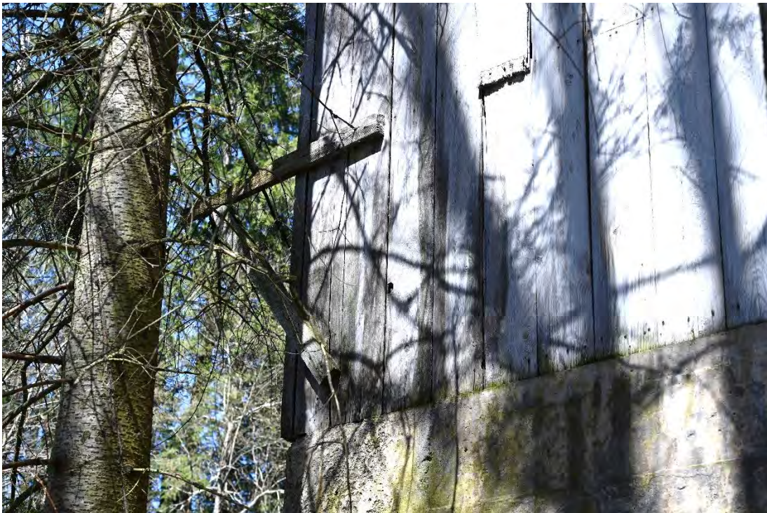
Figure 52. Close up view of bracket on back of gate house structure.
