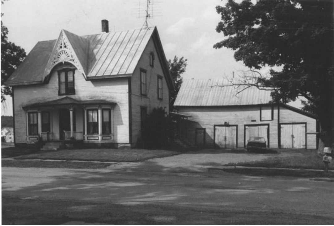
Figure 85. View northwest of a house along the north side of St. Albans Street (1984).
