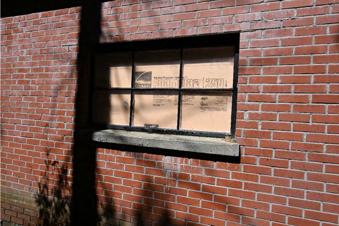
Figure 62. View southwest of window in the rear side of Well House #2.
