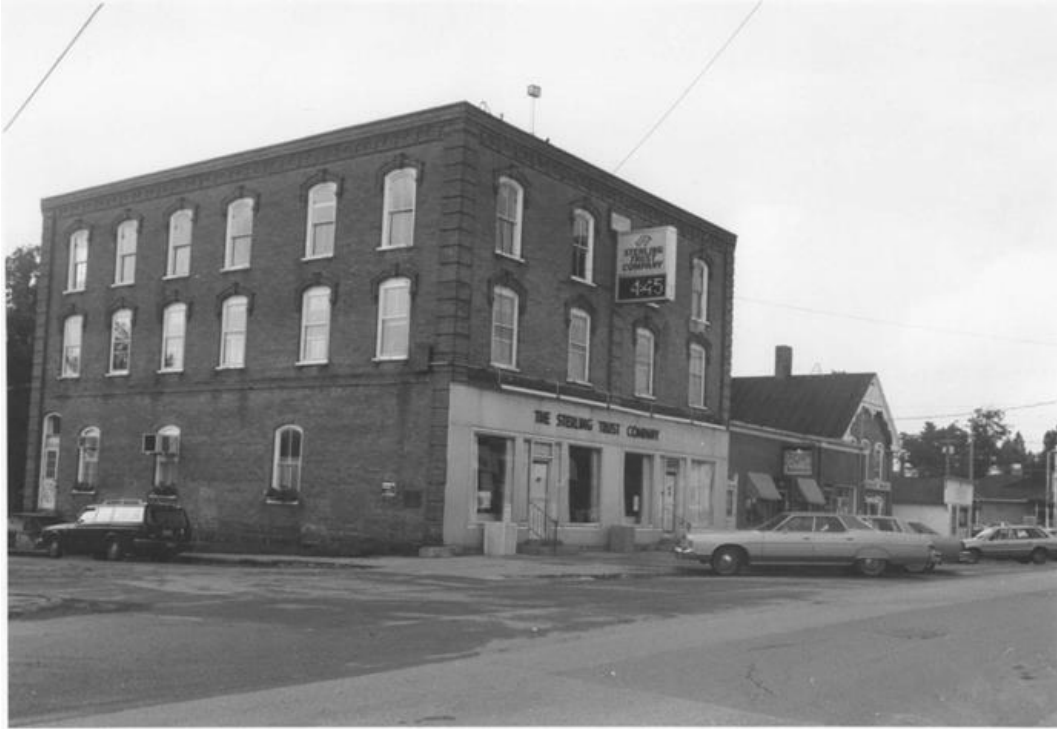
Figure 77. View northwest along Main Street (1984).
