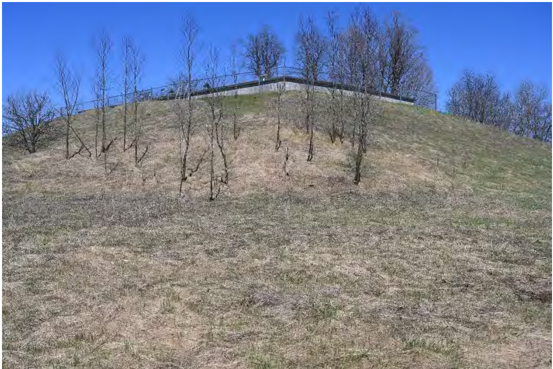
Figure 66. View northeast of the Concrete Reservoir.
