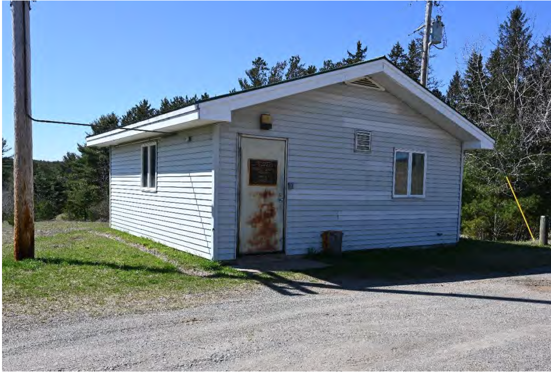
Figure 63. View northwest of the Chemical Feed Building.
