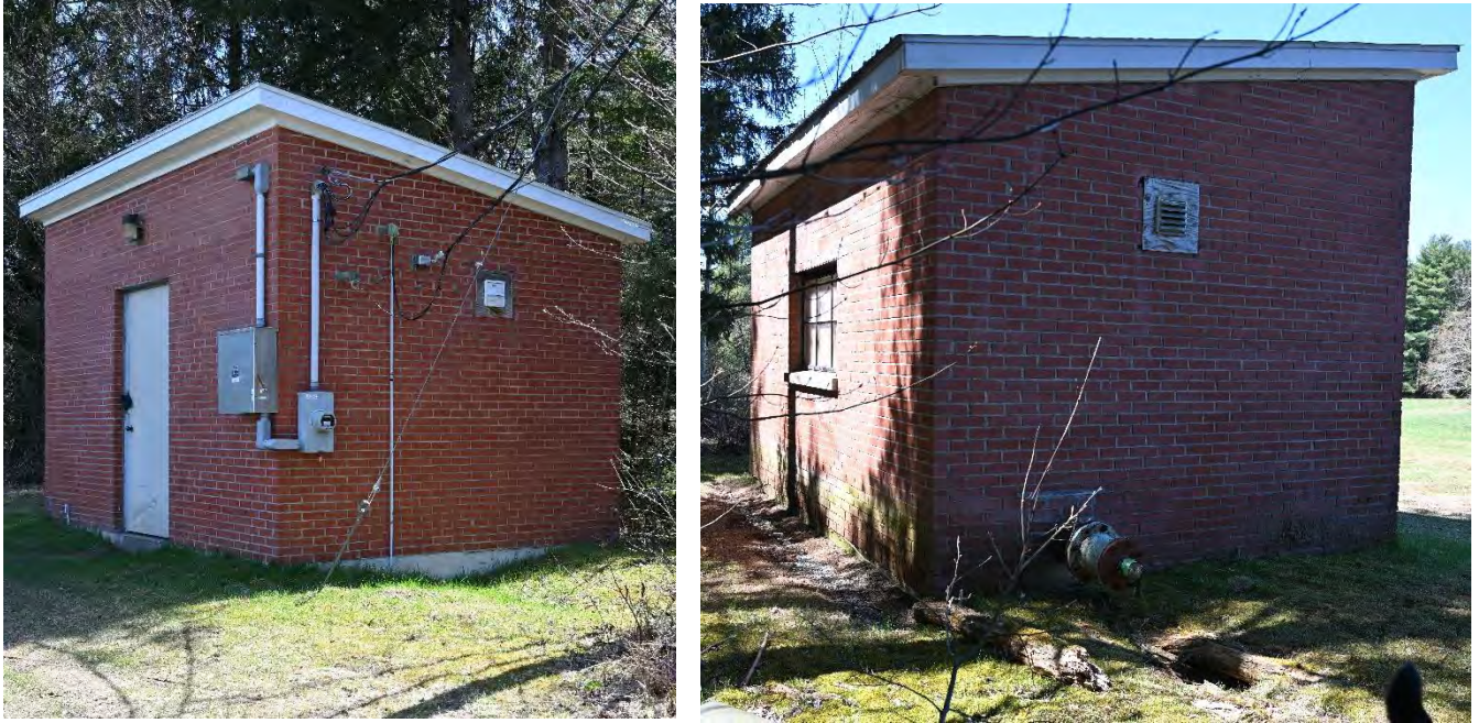
Figure 61. View northeast (left) and southwest (right) of Well House #2.
