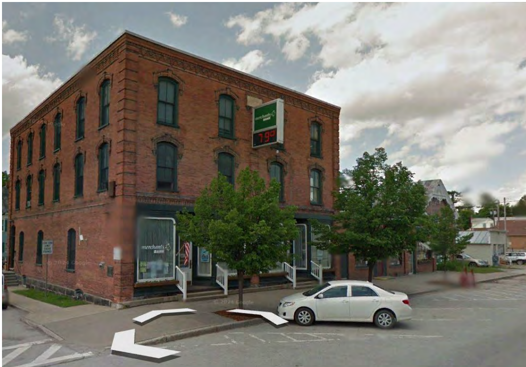
Figure 78. Google Earth view along Main Street (2012).
