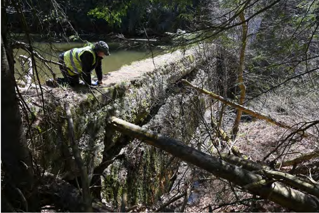
View northeast of the Trout Brook Reservoir Dam
