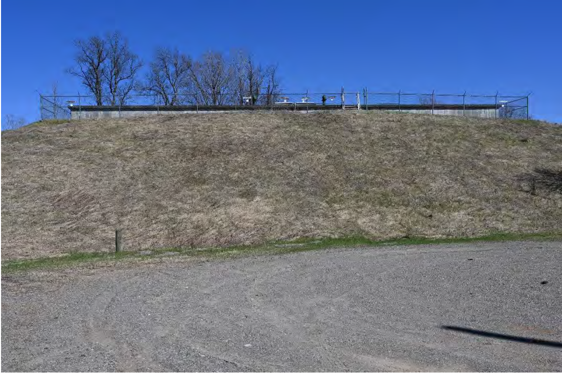
Figure 65. View east of the Concrete Reservoir.
