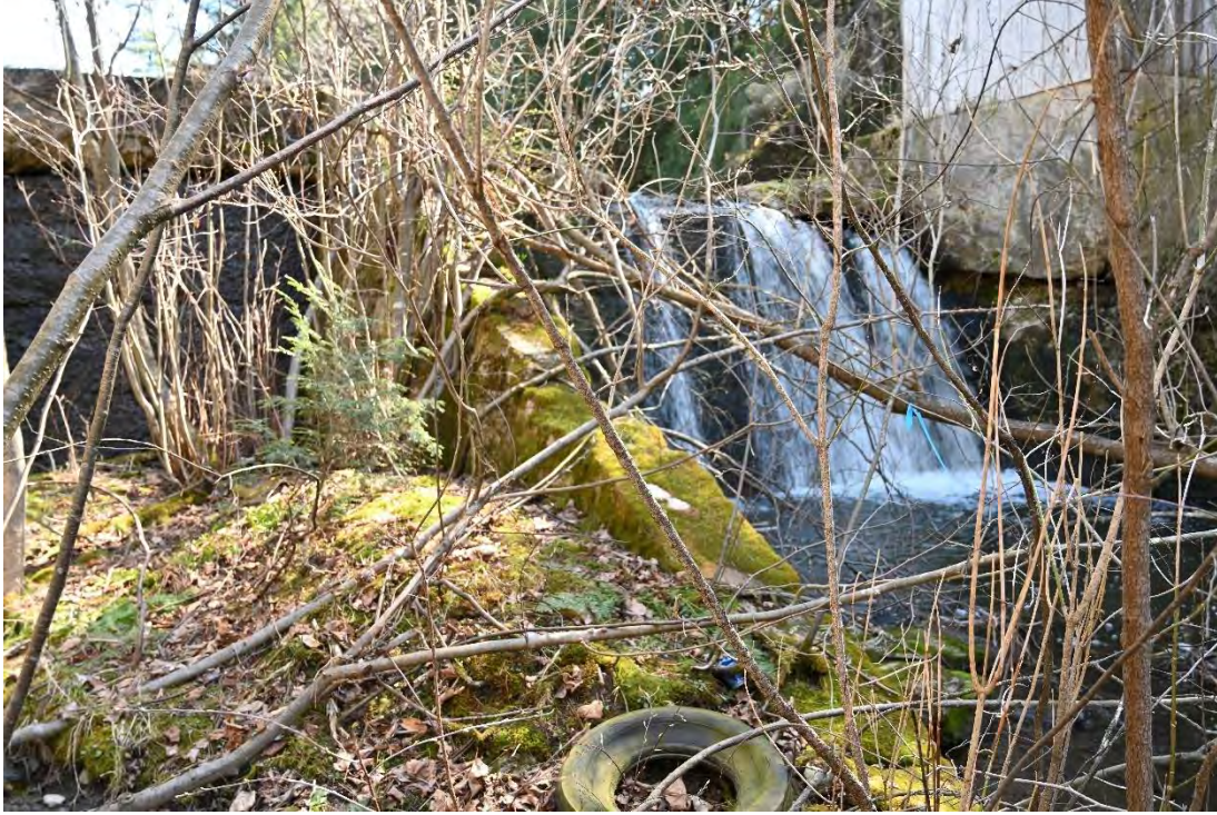
Figure 37. View of the Trout Reservoir Dam, looking northeast.
