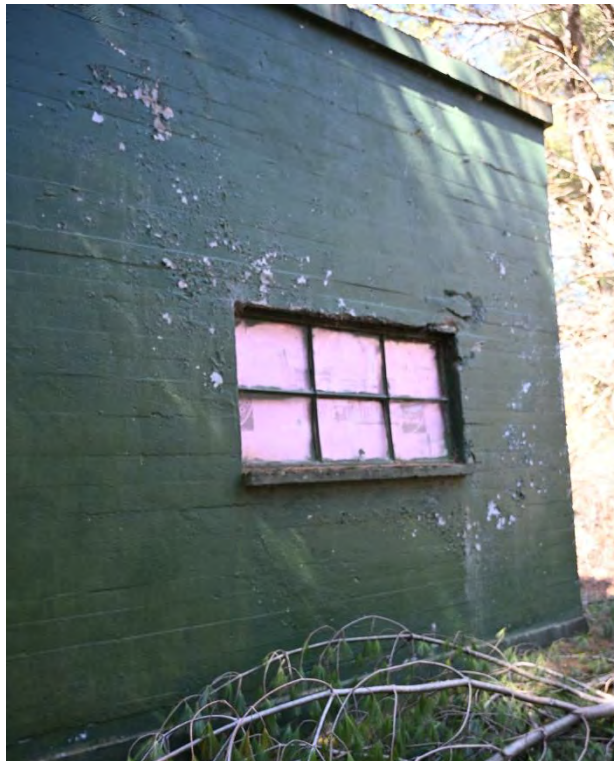
Figure 60. View northwest of the rear side of Well House #1.
