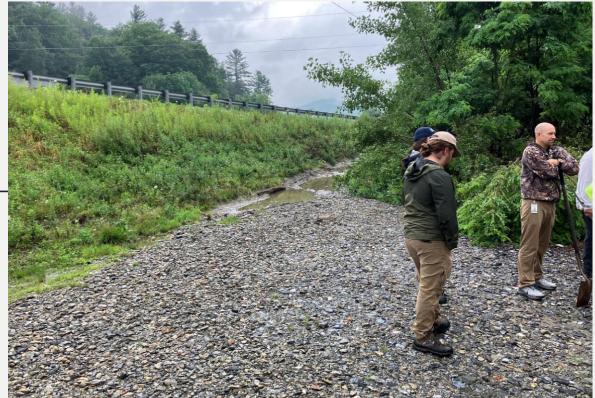
Post July 2023 flood, Dorothy Smith Access Area -Lower Access Area
