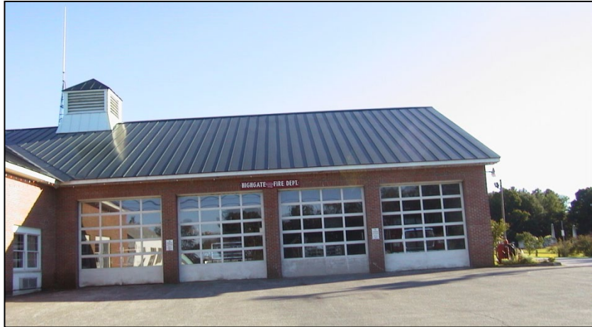
Highgate Fire Department
