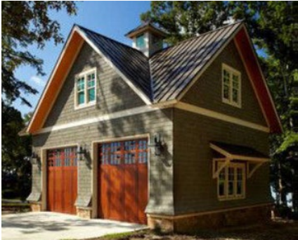
Above: floor plan of a one-bedroom Accessory Dwelling Unit (ADU) above a detached garage. Left: Image of detached garage with ADU.
