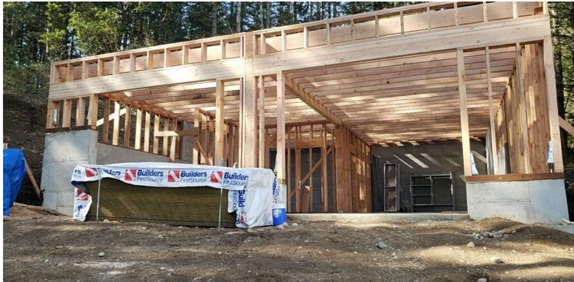
Attached new garage and ADU under construction
