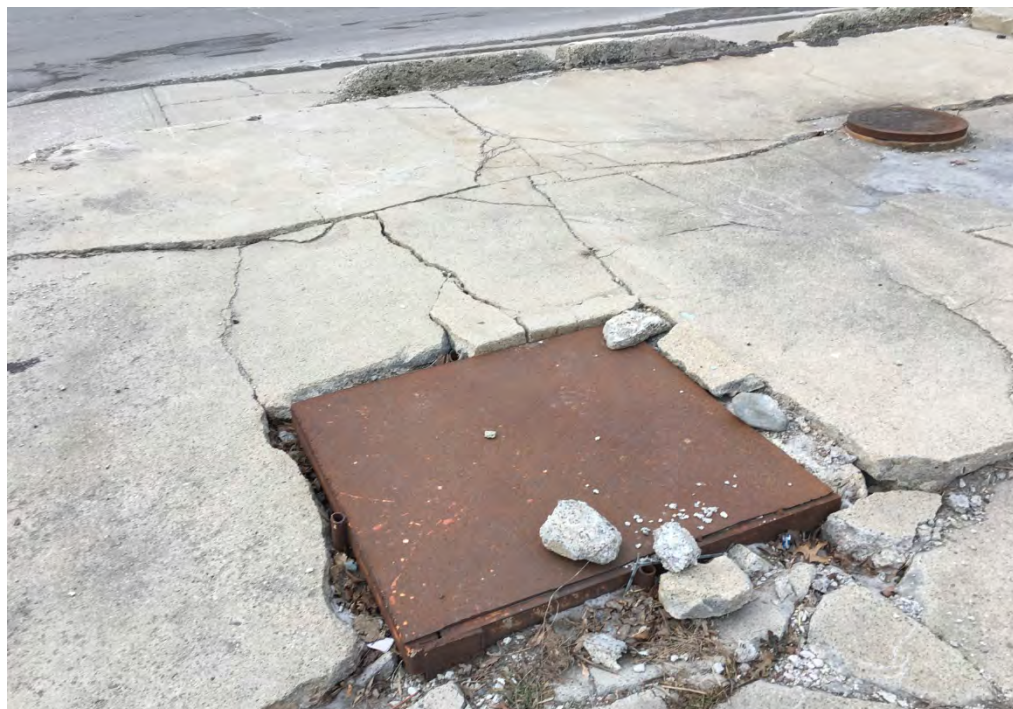
Photo 27: 25 Stebbins Street: Sewer features were observed within the concrete slab of 25 Stebbins Street. Photo taken facing northwest by Sanborn Head on January 10, 2017.
