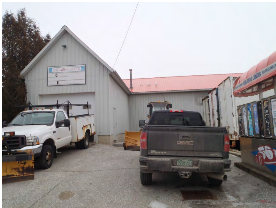
Photo 40: 21 Stebbins Street: The exterior of the former car wash building. Photo taken facing east by Sanborn Head on January 10, 2017.
