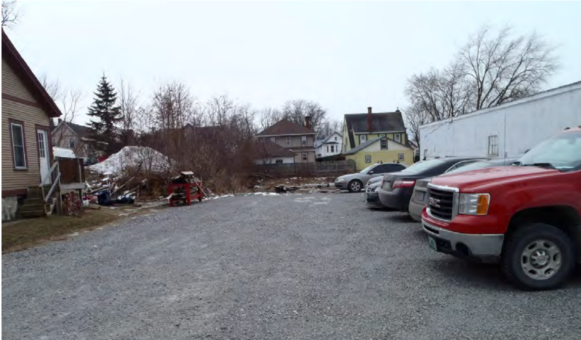
Photo 1: 12 Stebbins Street: View of the property located at 12 Stebbins Street. Photo taken facing south by Sanborn Head on January 10, 2017.
